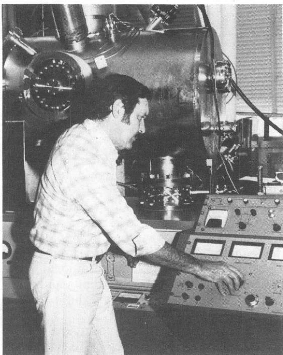
FOR TOKOMAK — Art Mullendore (5834) prepares to run test in combined environment test chamber upon coated materials samples. The coated materials are under test as possible first wall materials in tokamak fusion devices at Princeton and Oak Ridge.
